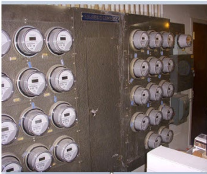
Figure 2. Ganged Meter Sockets
