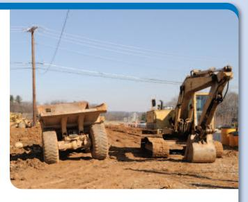
high-voltage lines. The watch's only duties should be observing the work and communicating with the operator to ensure the equipment never violates the Circle of Safety.
