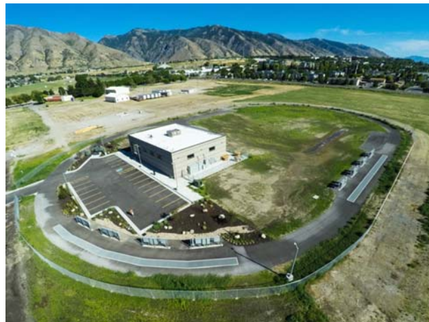
Figure 4. USU EVR capabilities include 750 kW utility, 4,800 sq ft dual high bay, quarter mile test track, L2 and 50kW DC fast charging, DC & AC microgrid, 100 kWh on-site energy storage, and 120kW solar array.
