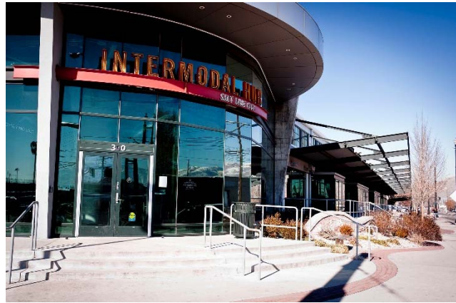
Figure 1. Utah Transit Authority Intermodal Hub in Salt Lake City.
