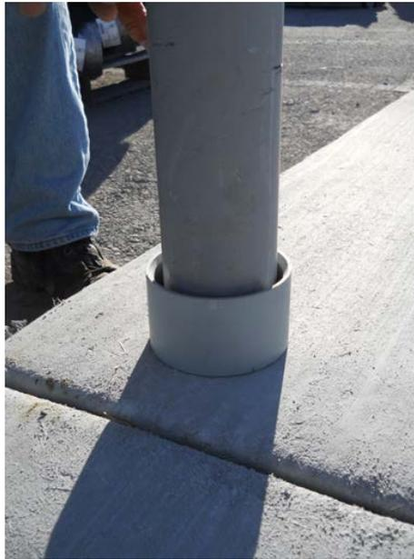
**Figure 24—Installing Conduit through Concrete**
