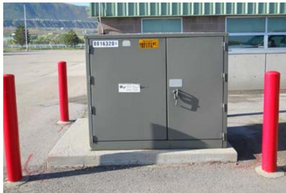
**Figure 40—Barrier Posts, Example**
