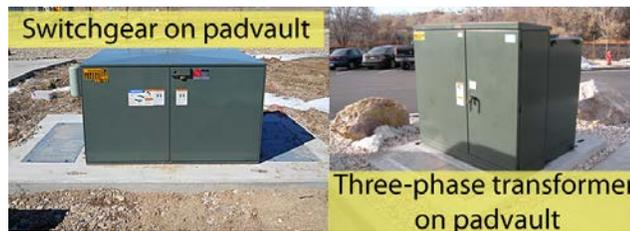
**Figure 63—Switchgear and Three-Phase Transformer on a Padvault**
