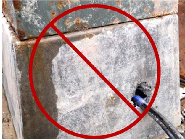
**Figure 53—Hole through the Side of a Fiberglass Box Pad**
