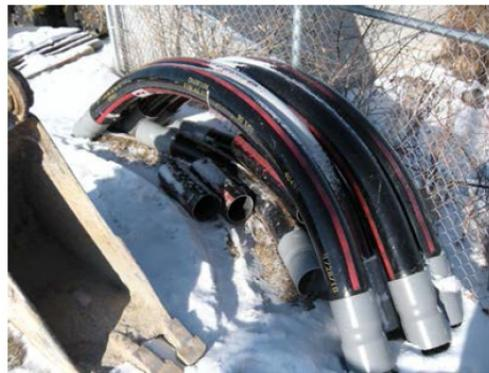
**Figure 19—Fiberglass Sweeps**
