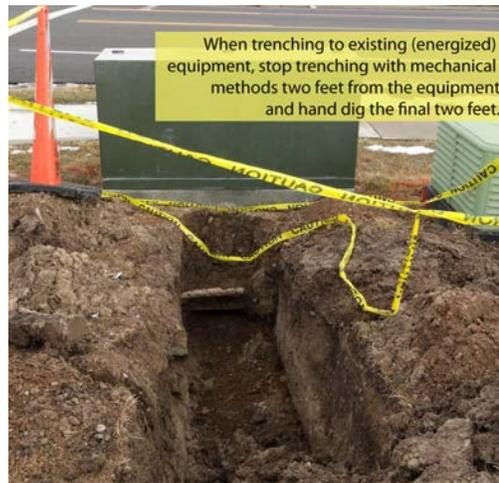
**Figure 5—Trench to Energized Equipment**
