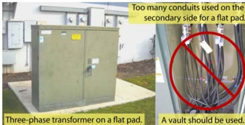
Figure 60—Three-Phase Transformer Flat Pad
