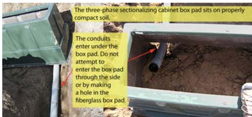
**Figure 52—Conduit Placement – Three-Phase Sectionalizing Cabinet**
