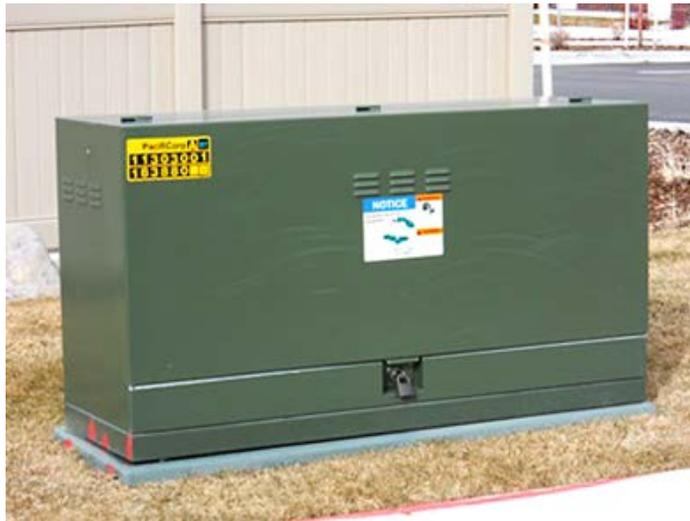
**Figure 48—Three-Phase Sectionalizing Cabinet**
