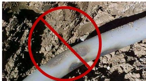
Figure 21—Field Altered Sweep – Damaged PVC
