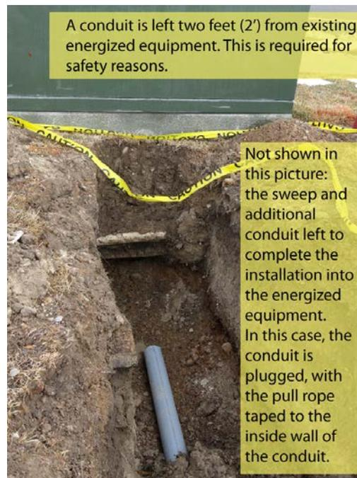
**Figure 23—Installing Conduit to Existing (Energized) Equipment**
