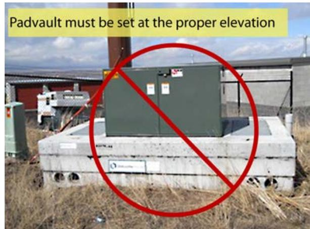
**Figure 66—Padvault Not Set at the Proper Elevation**
