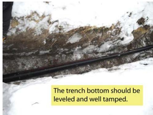
**Figure 13—Typical Primary Conductor Trench**
