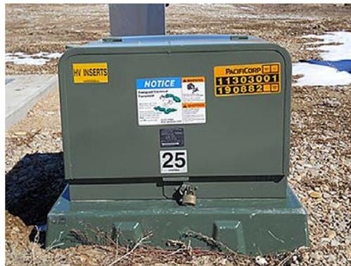
**Figure 54—Single-Phase Transformer**
