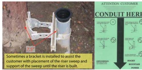
**Figure 31—Riser 7.5" from Pole, Bracket and Power Company Template**
