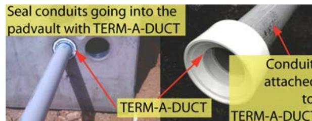
**Figure 68—TERM-A-DUCT Used for Conduit Entering the Padvault**
