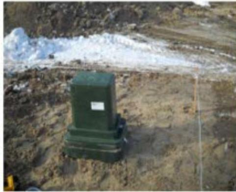
**Figure 70—Installed Secondary Box with Pedestal**
