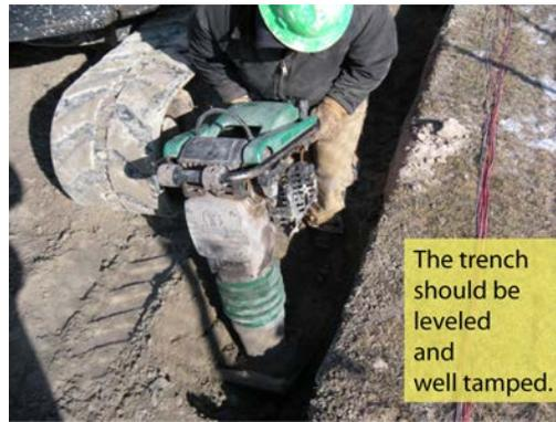
**Figure 14—Typical Conductor Trench**
