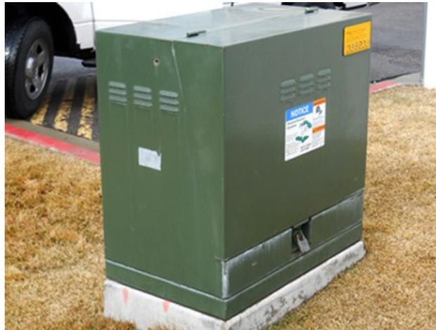
**Figure 43—Single-Phase Sectionalizing Cabinet**
