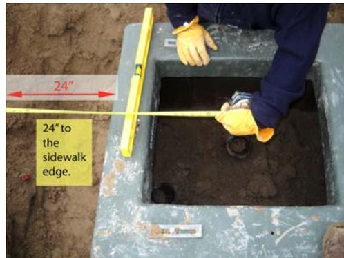
**Figure 36—Positioning of a Box Pad**
