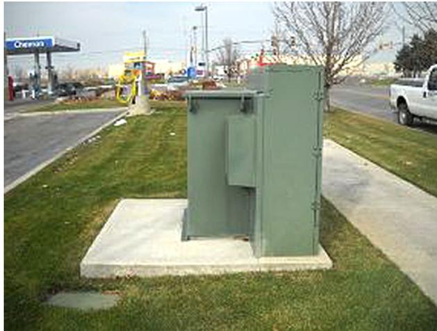
Figure 59—Three-Phase Transformer on a Flat Pad
