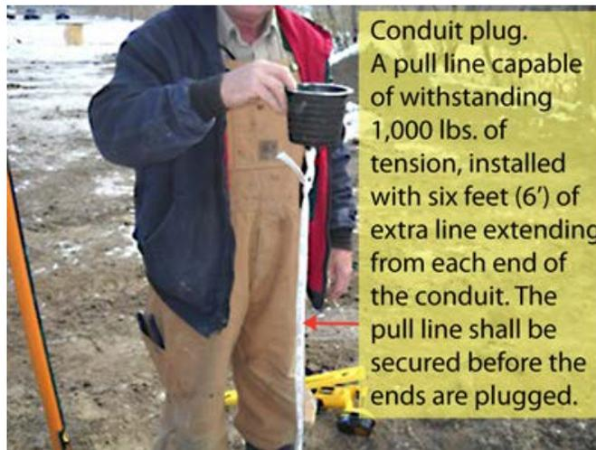
**Figure 27—Conduit Plug and Pull Line**
