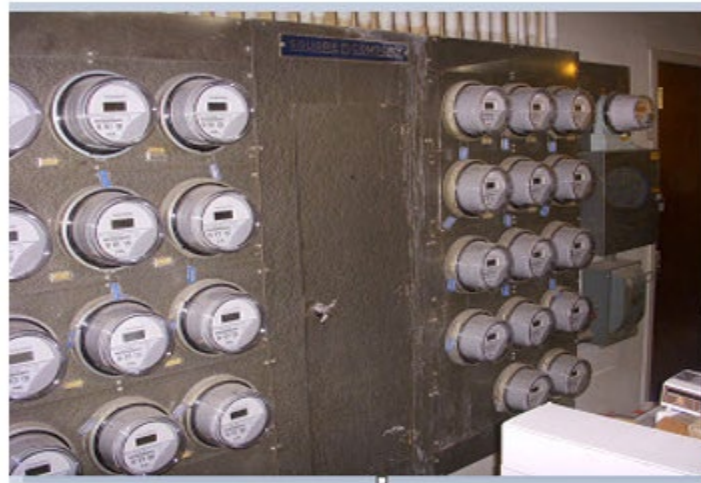
Figure 3. Ringless meter base.
