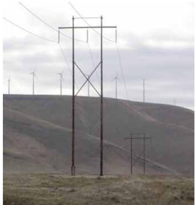
A typical wood pole 230kV structure that will be used in the new transmission line project.
