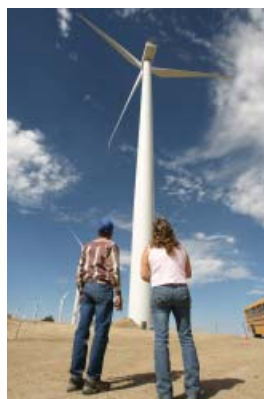
Glenrock wind farm
