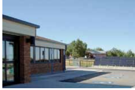
Solar panels sit adjacent to the Meals on Wheels building in Casper
